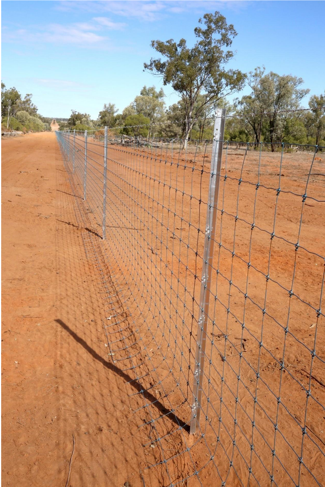
Cluster exclusion fencing for wild dog control © The State of Queensland 2020
